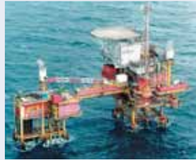
Four Crude oil pumps in the North Sea (Dual Voltage 2300-3300V / 160A)
