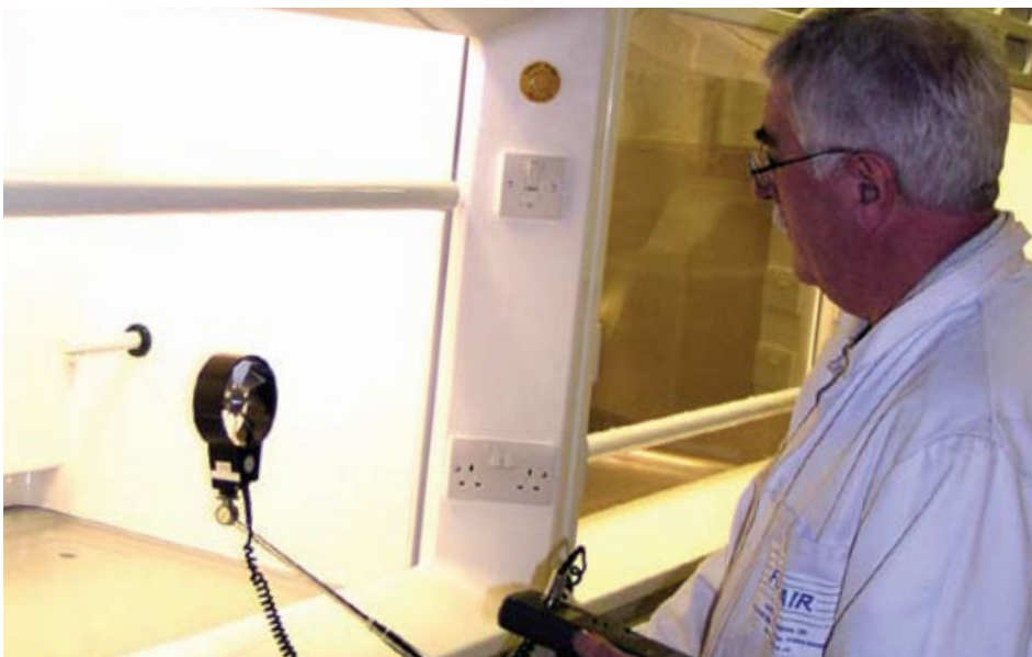
● Checking the fume cupboard airflow
